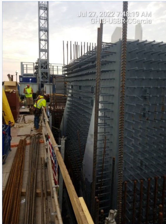
First anchor box installation July 2022 US
