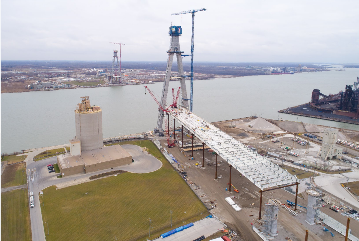
Backspan deck February 23, 2023, US
