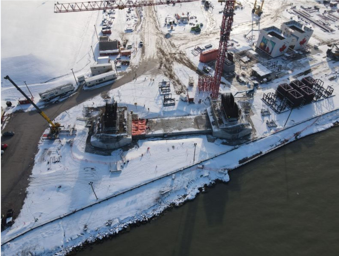
Tower footings and tie-beam Canada
