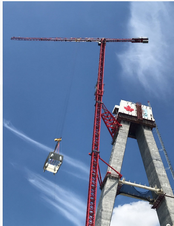
First anchor box installation August 2022 Canada
