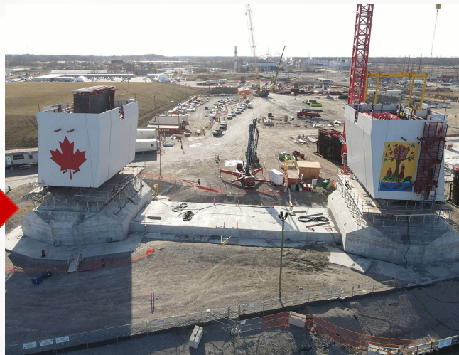
Canadian Tower Footing with Tie beam (2021-02-12)
