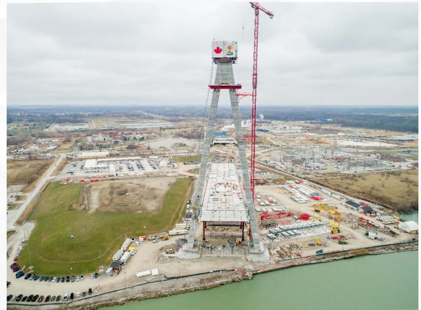
Canadian towers February 23, 2023
