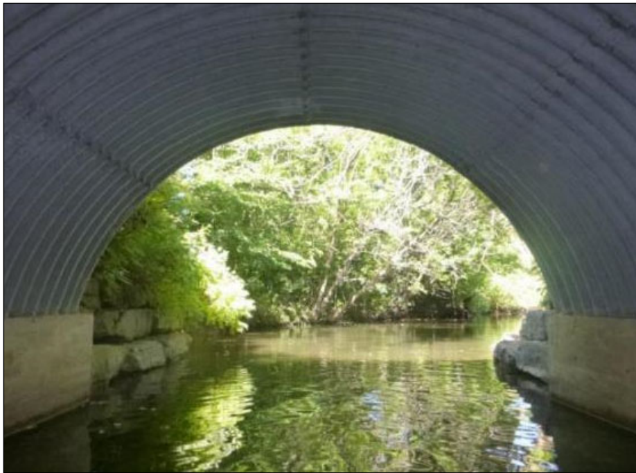
Existing Arch on Spread Footings
