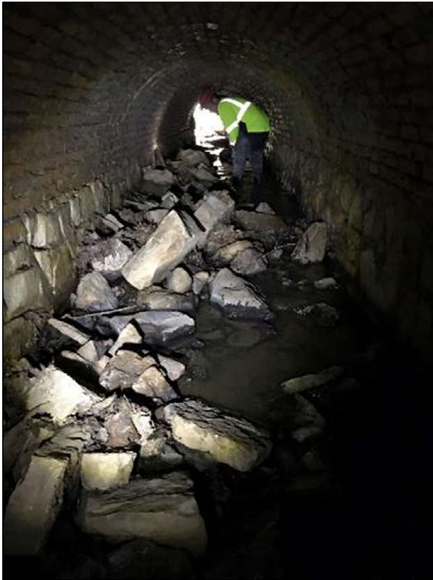
Initial Culvert Conditions
