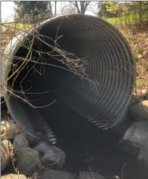
Existing Culvert Condition
