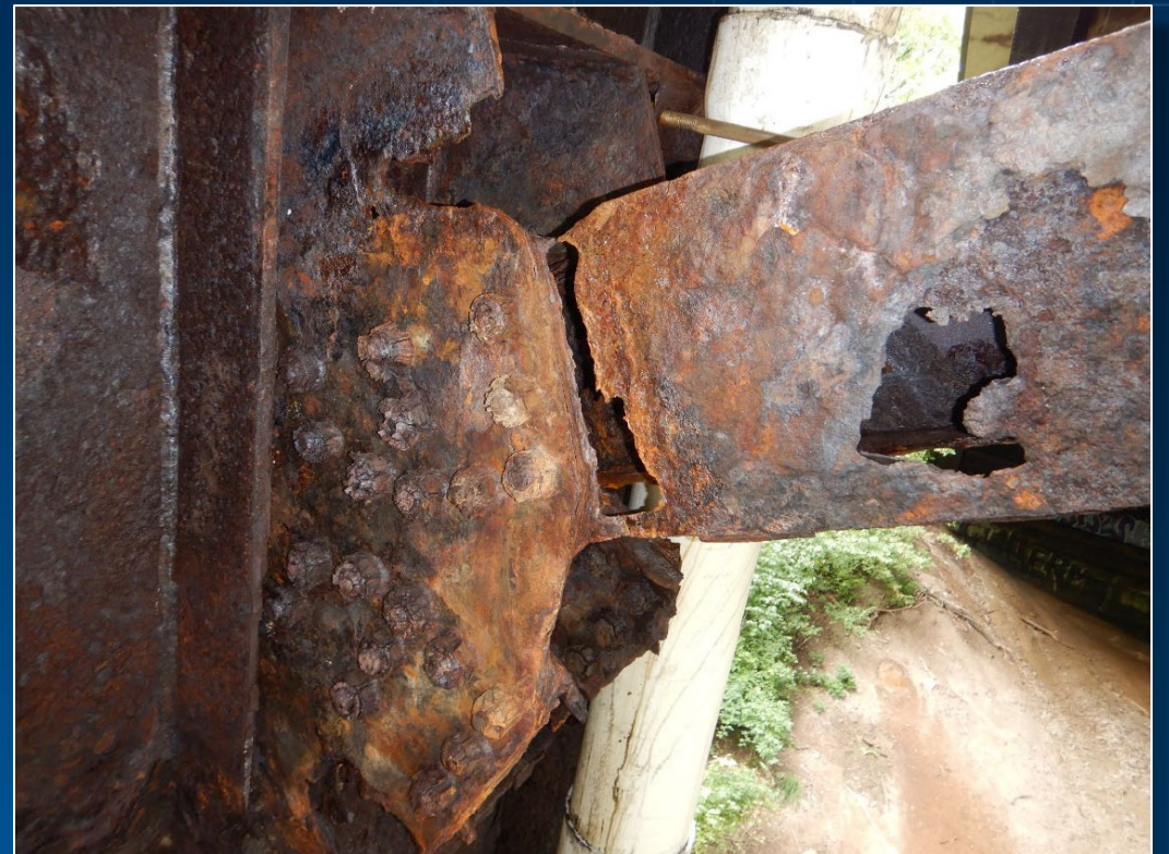
Source: 2021 inspection report
