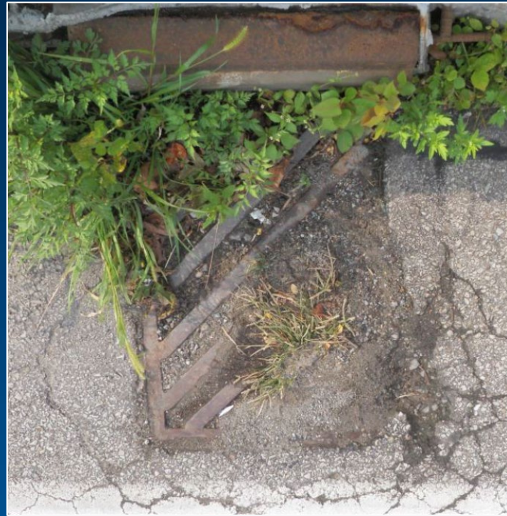
Source: 2017 inspection report
