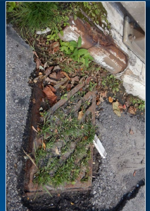
Source: 2021 inspection report
