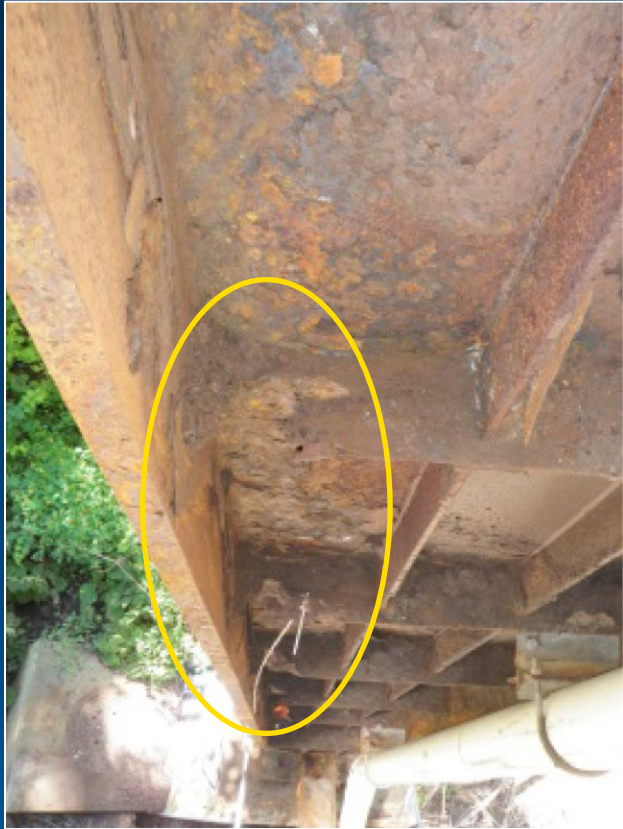
Source: 2013 inspection report
