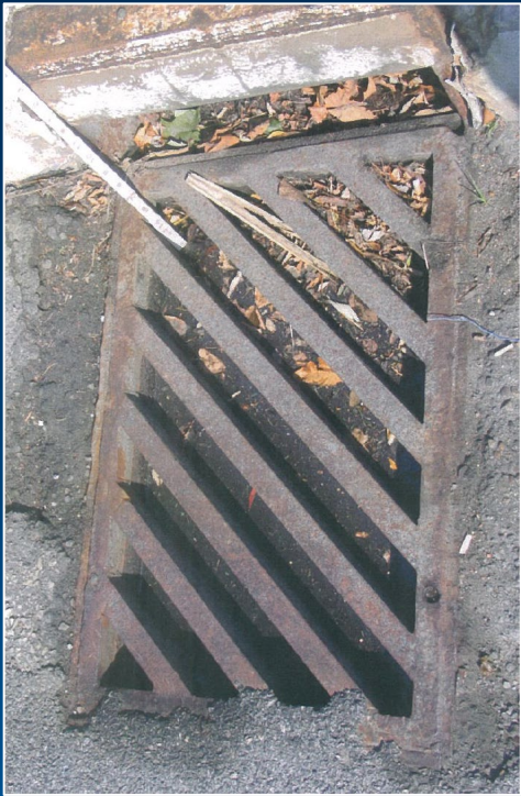
Source: 2005 inspection report
