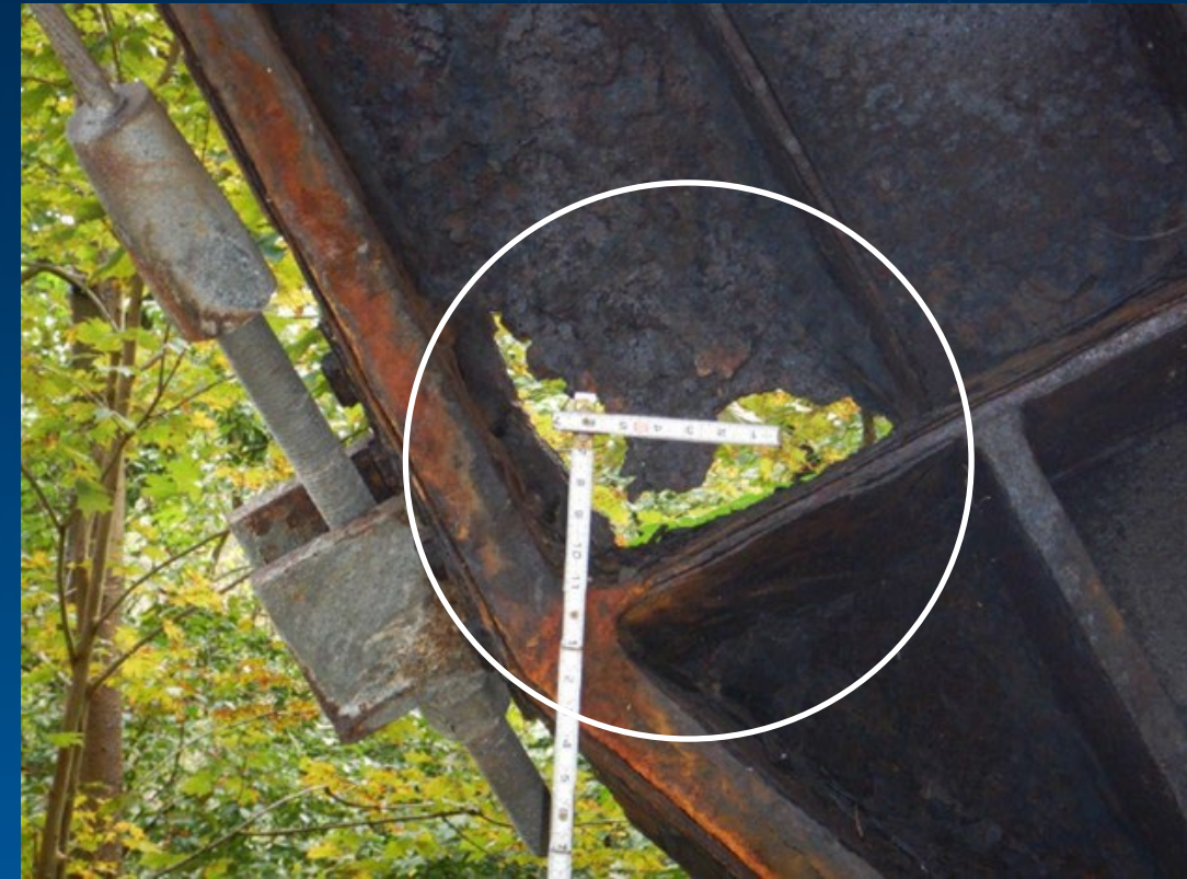
Source: 2021 inspection report
