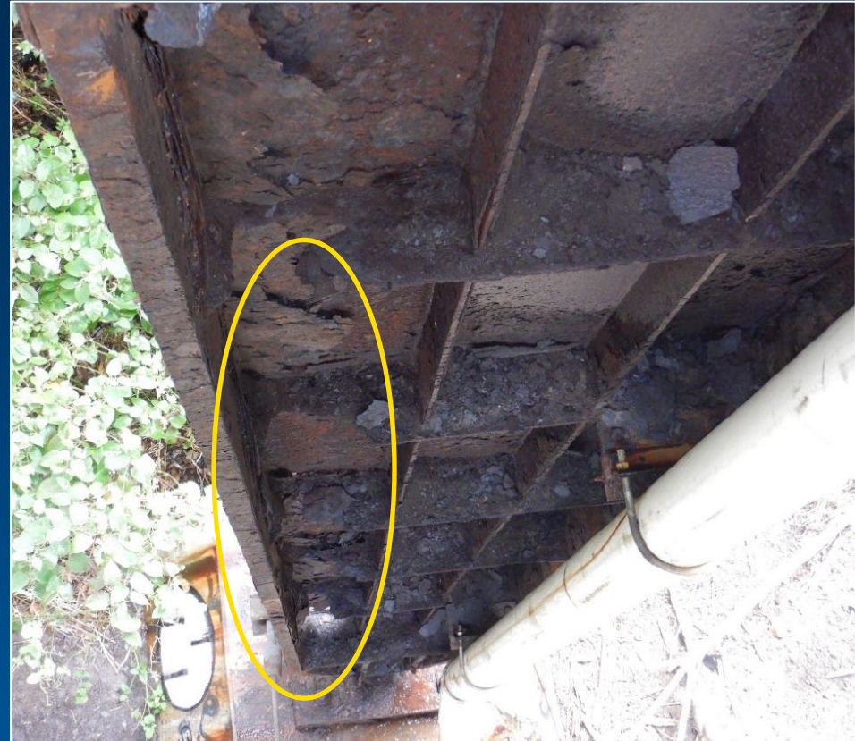
Source: 2021 inspection report
