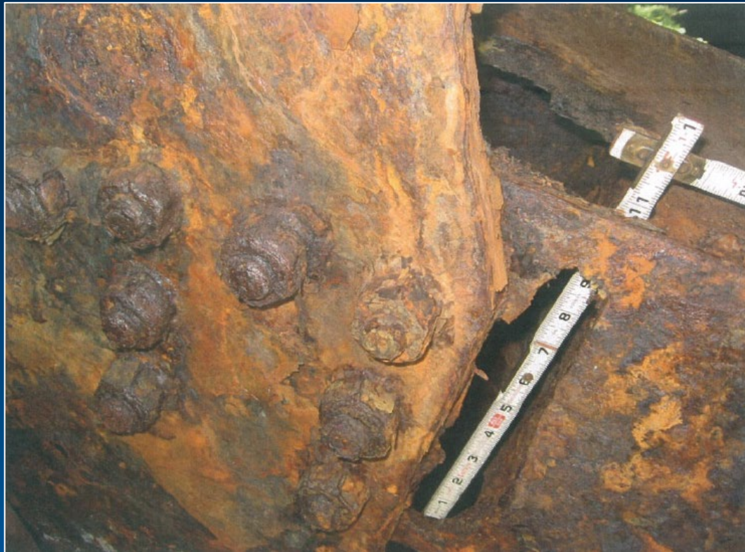
Source: 2005 inspection report
