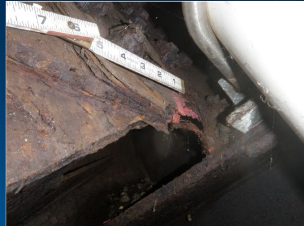
Source: 2015 inspection report
