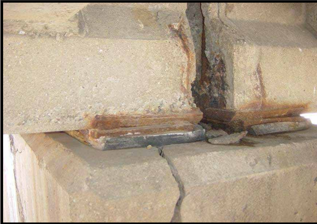
Loss of Bearing Area
