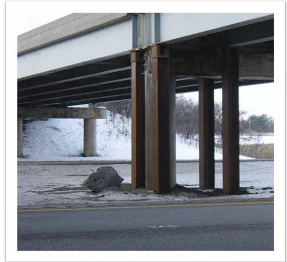
Full Height Temporary Support
