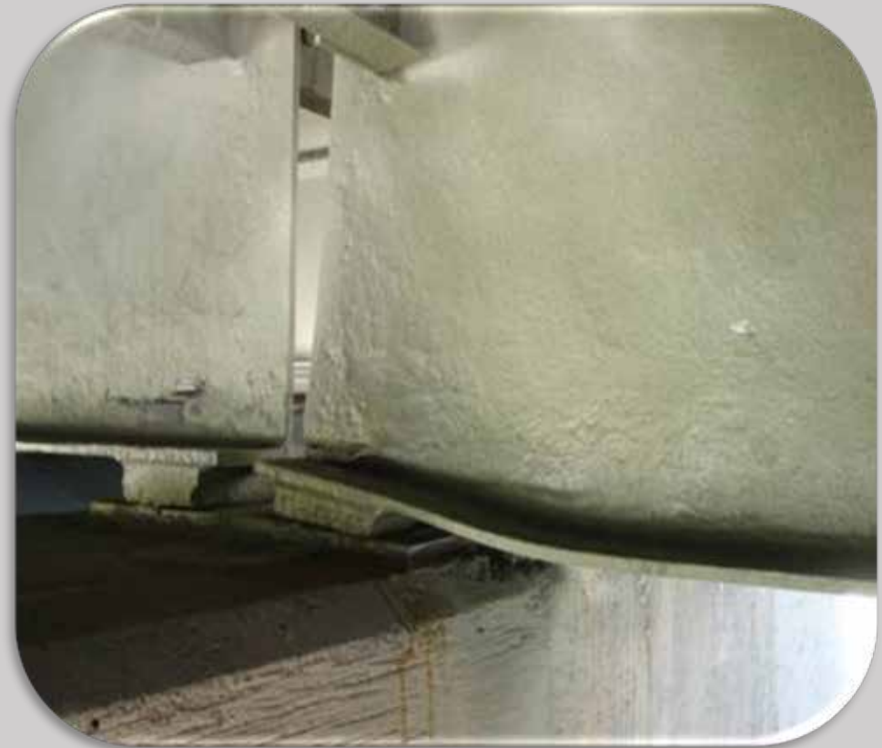
Buckled Beam Ends
