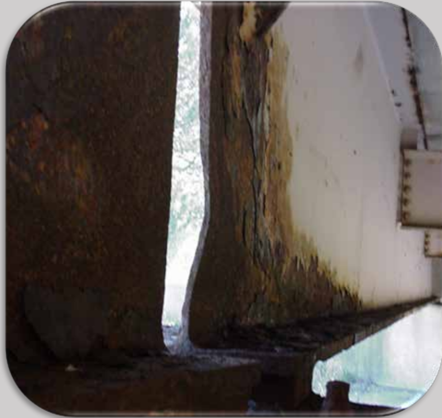
Buckled Beam Ends
