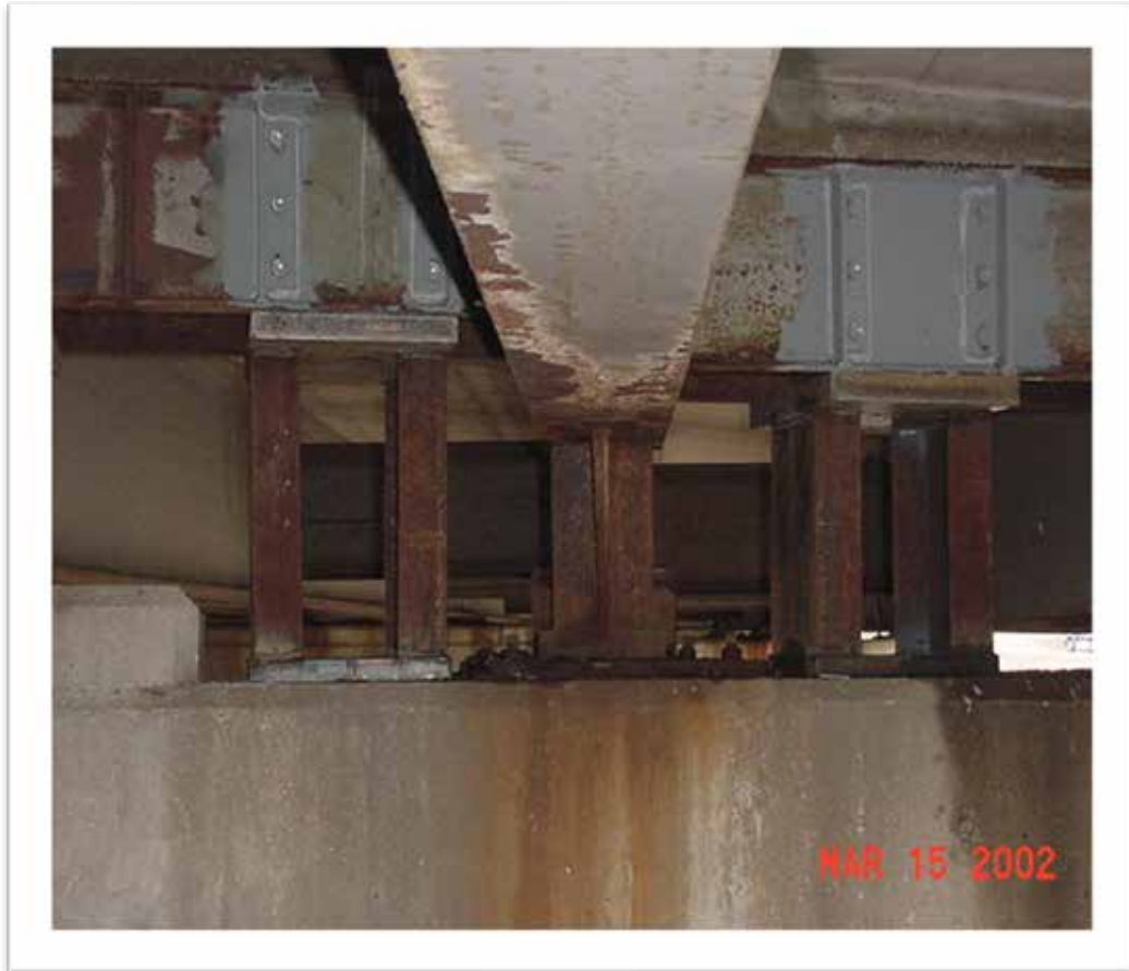
Short Height Temporary Support
