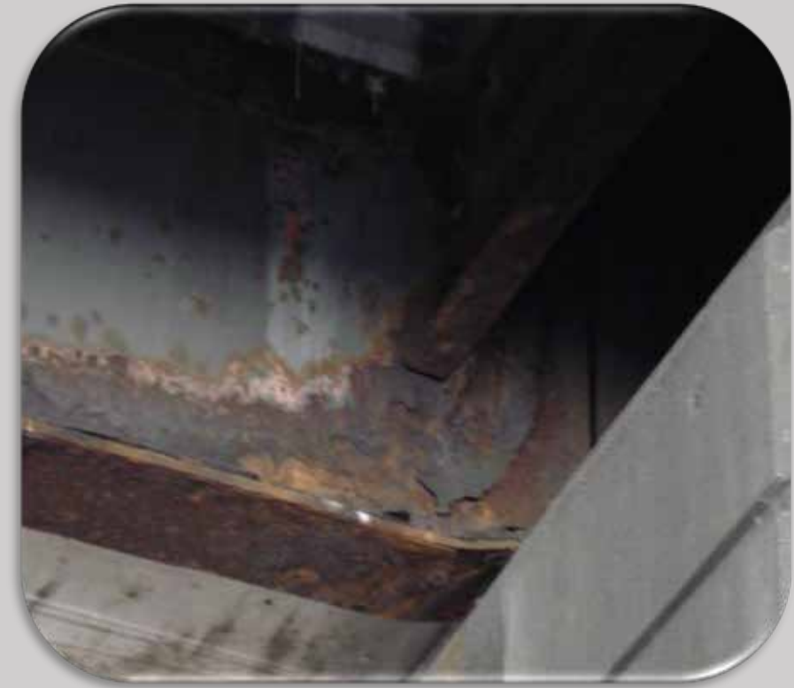
Buckled Beam End due
