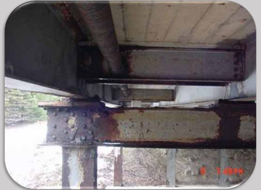
Cracked, holes/buckled beam and pier cap (corrosion)
