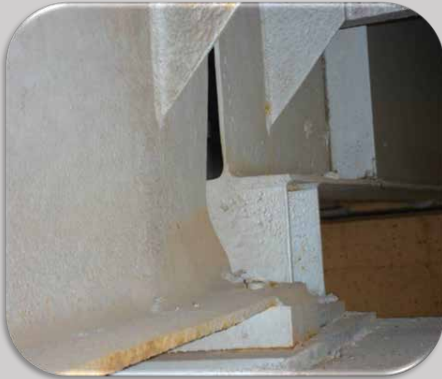
Buckled Beam End due
