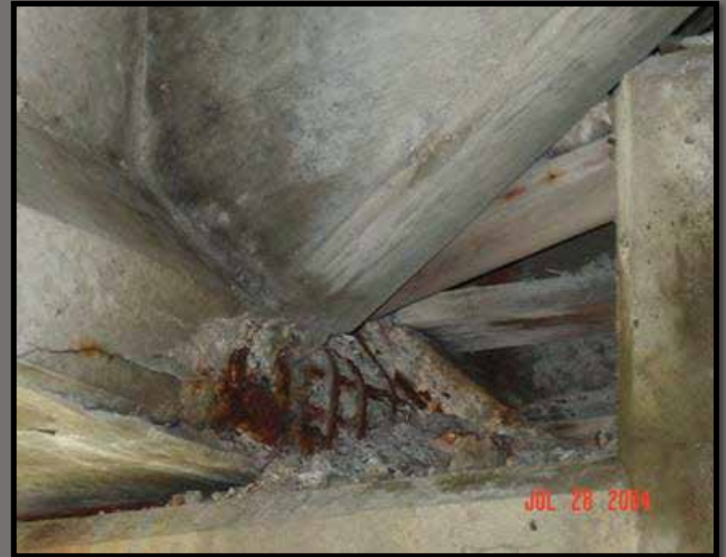
Loss of Bearing Area
