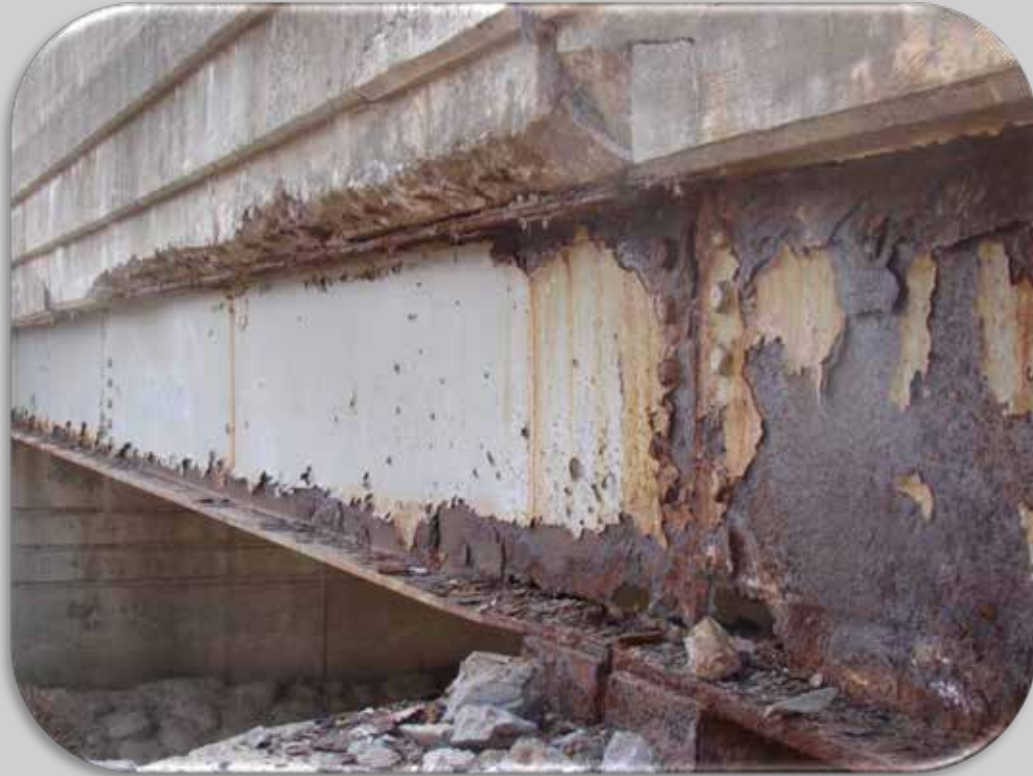
Cracked, holes/buckled beam and pier cap (corrosion)
