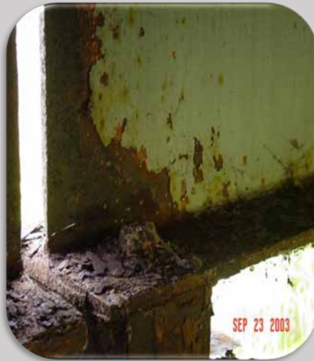
Cracked Beam Ends
