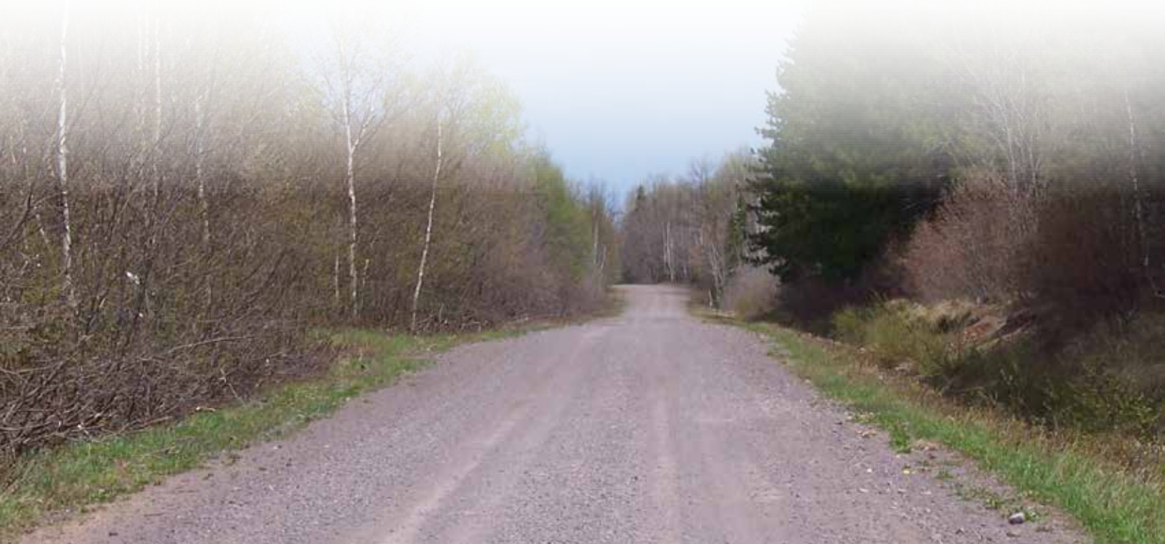
Road with an IBR number of 8, having fair surface width, good drainage adequacy, and good structural adequacy
