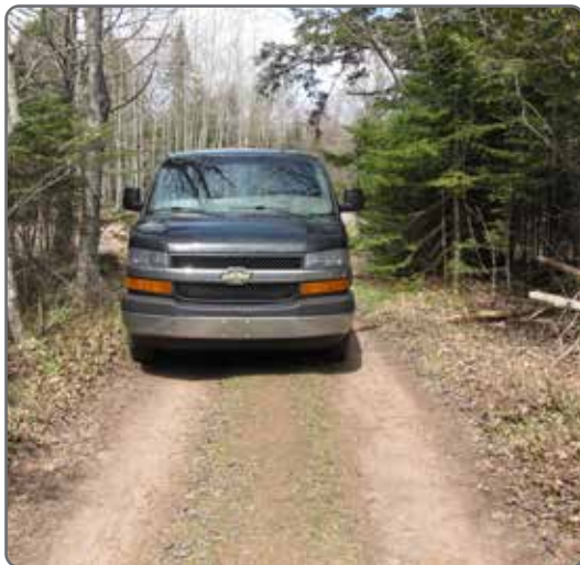
Figure 4: Even if an unpaved road appears to have good surface condition, it is still likely to perform poorly without proper drainage.
