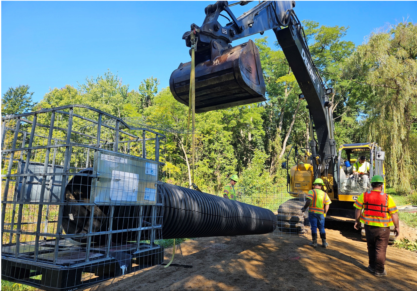
Washtenaw County Road Commission – Excavator Hold Up/Beaver Mitigation
